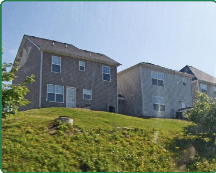
Recently-built single-family homes in Palmetto
