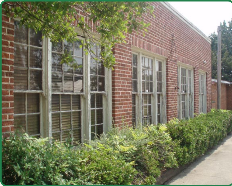
Palmetto's historic mill area was identified as a rehabilitation opportunity
