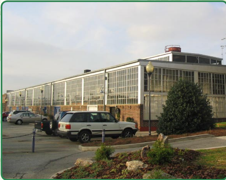
Local stakeholders cited examples such as King Plow Arts Center when envisioning the future of the Historic Mill site
