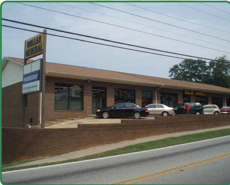
Commercial building on Main Street
