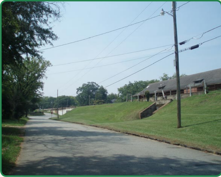
The excess land along the west side of Cobb street could accommodate a dedicated bicycle facility and sidewalks
