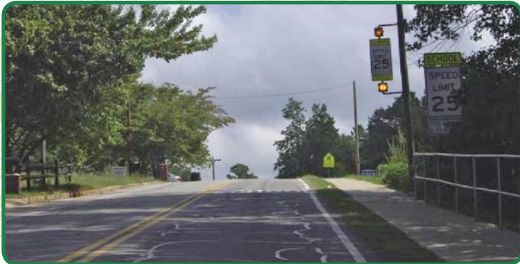
School zone traffic control Carlton Rd.
