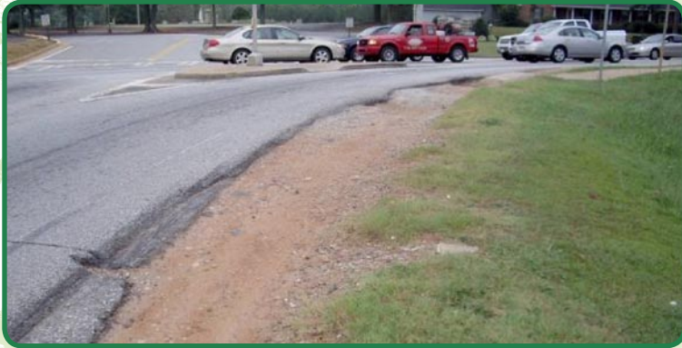
Roadway at Roosevelt Hwy./Cascade Palmetto Hwy shows sidewalk ending abruptly into a low, soft shoulder with evidence of vehicle off-tracking
