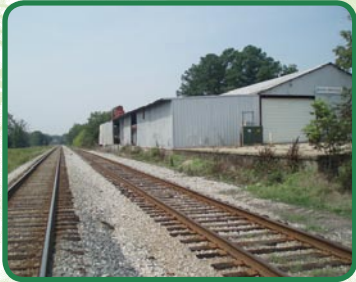
Spurlin - industrial site along rail-road
