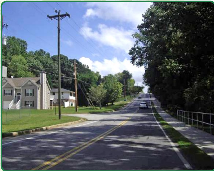
Carlton Road's wide lanes and straight alignment likely contribute to high vehicle speeds.
