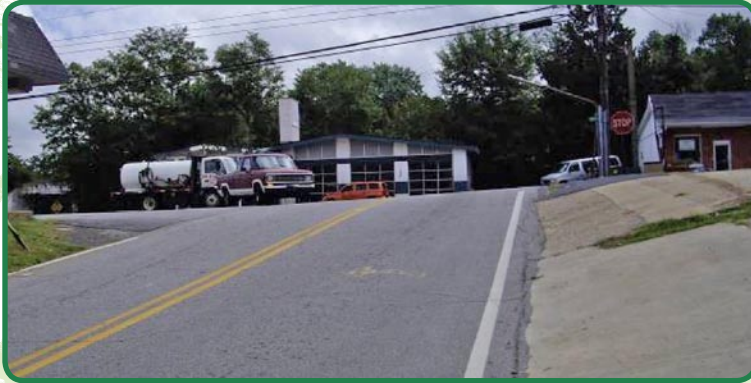
Menefee St. approach to Main St. has a steep grade.
